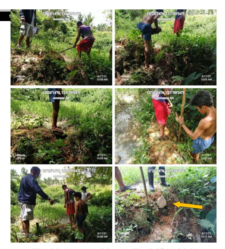
As an initial step, the inspection team recommends the owner to seal the opening (yellow arrow) wherein it was immediately done. Also, the owner committed to add additional height (sacks of soil) of the levee of the pond and to revive its former small fishpond.
