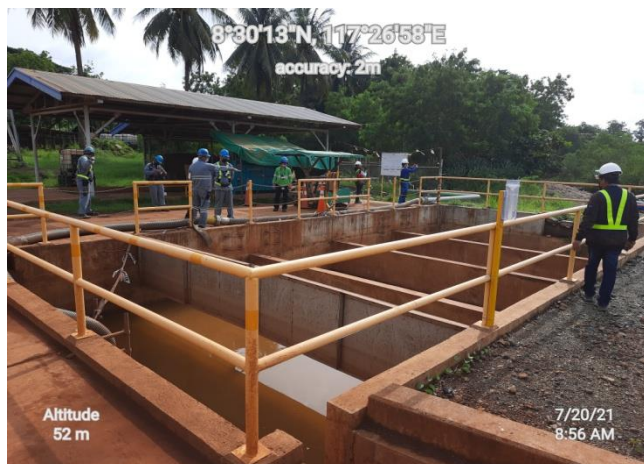
Maintained Silt Collector Sump
