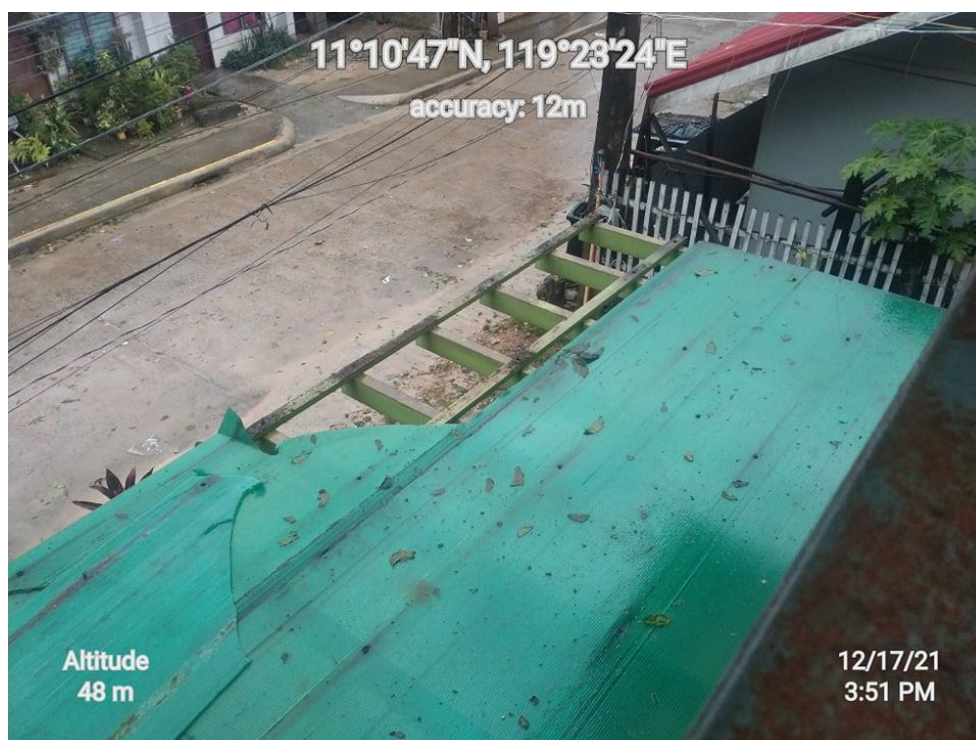
Partially damaged polycarbonate roof of the PAMO-ENTMRPA located along Calle Real, Bgy. Masagana, El Nido, Palawan
