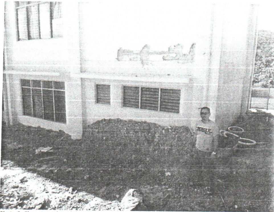
Photo 3. Closest portion of the Annex building to the slope where a previous landslide has encroached up to 2 meters of the building.
