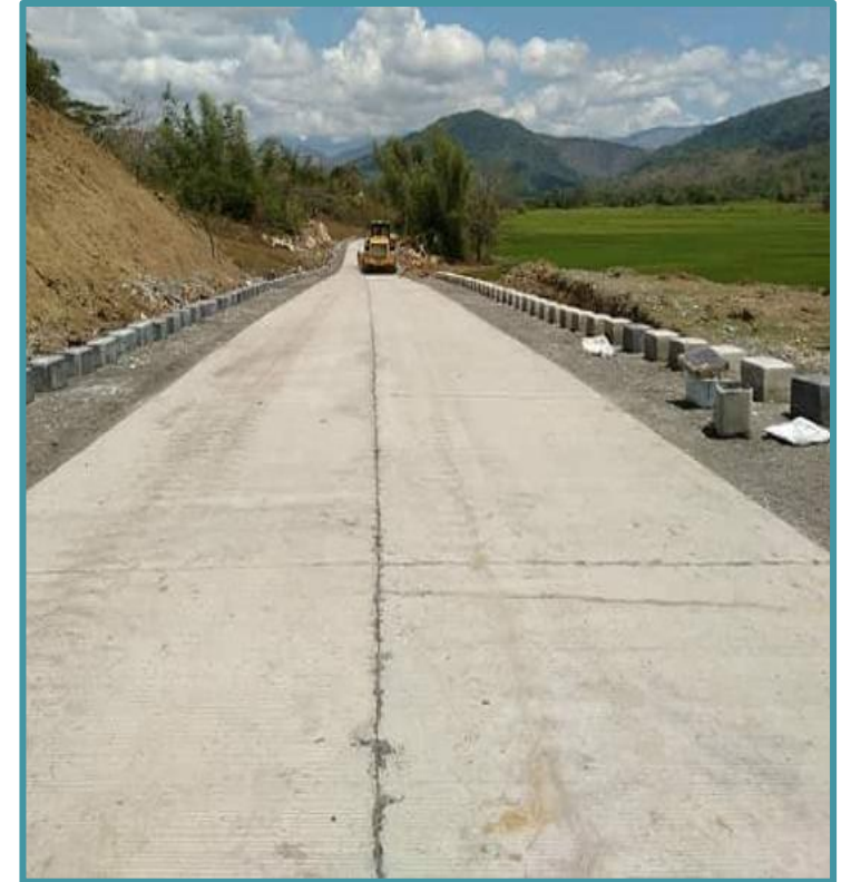
Farm-to-Market Road, Brgy. Monteclaro, San Jose, Occidental Mindoro
