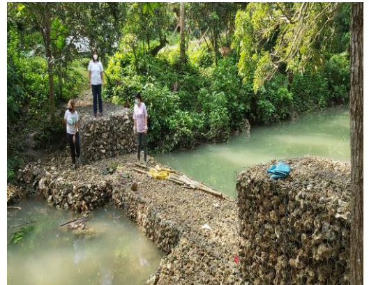
Gabion check dams under the BBB Task Force Project of typhoon hit provinces
