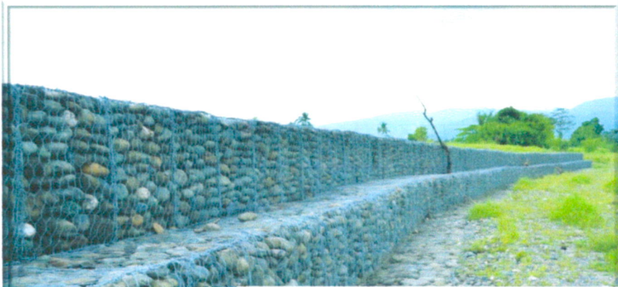
INFRASTRUCTURE OF GABION DIKE OF MAG- ASAWANG TUBIG AT VILLA CERVEZA VICTORIA
