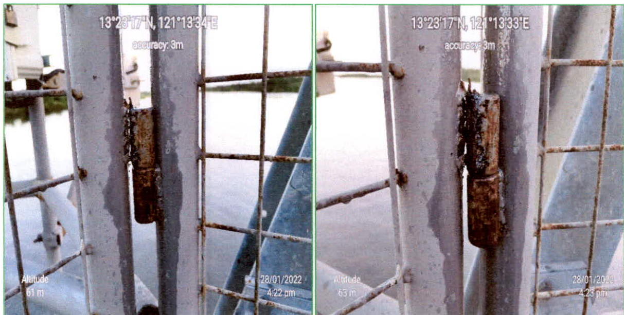
Figures 13: Pictures showing the broken welding of the middle hinge of the gate of the AWLS
