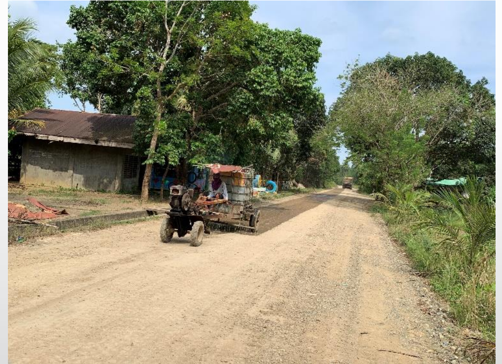
Water spraying of the hauling road
