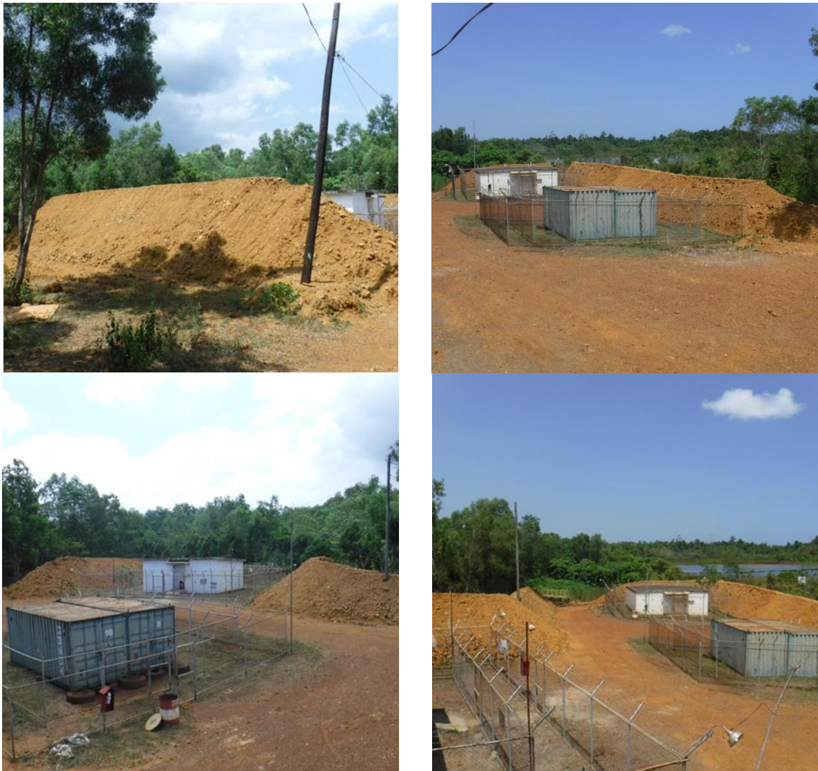
Plate 3. Constructed berm at the Magazine area
