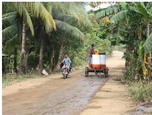
Plate 1. Water spraying of the hauling road
