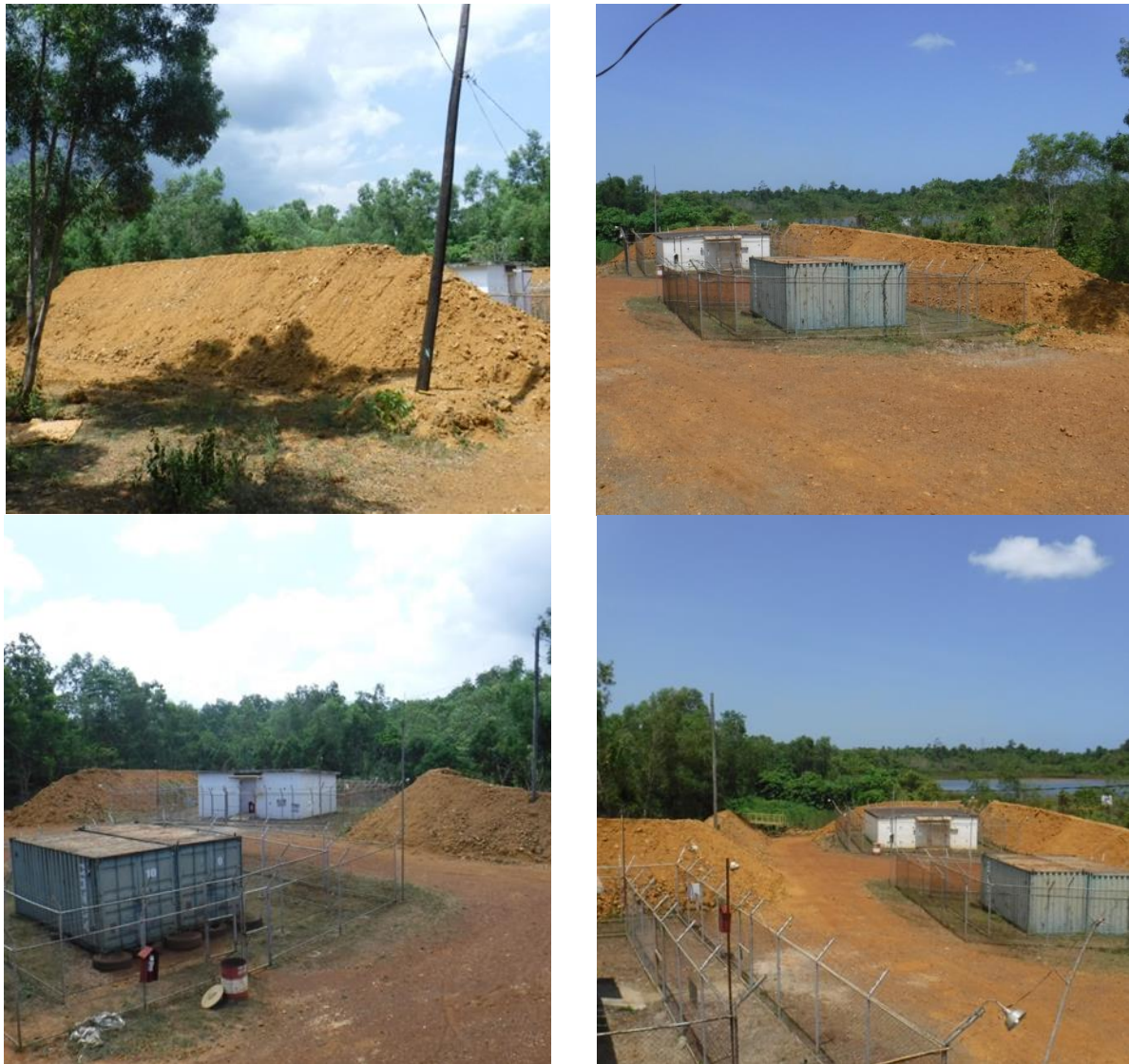
Plate 3. Constructed berm at the Magazine area
