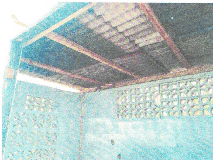
Installed temporary roof of generator house
