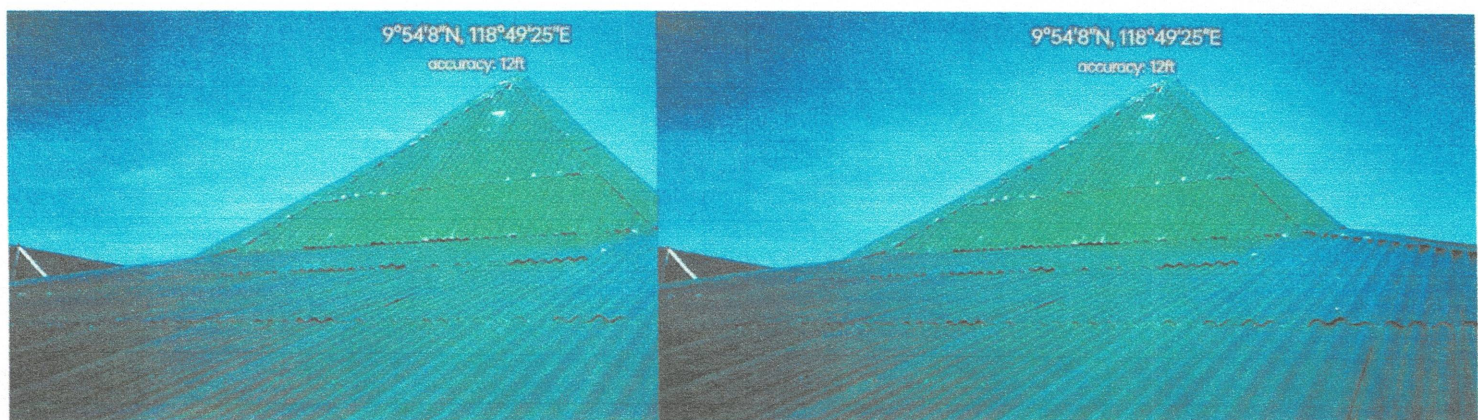
Photos of the repaired and newly painted roof of Admin Building
