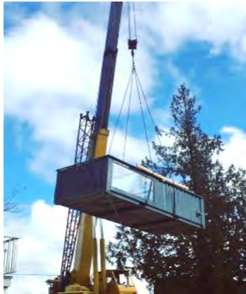
MODULAR POOL INSTALLATION
