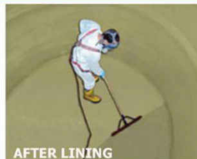
AFTER LINING Chemical Storage Tank after being re-lined with fiberglass.
