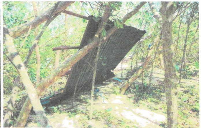
Photo of damaged Generator House (left) and photo of detached roof from Generator house (right)
