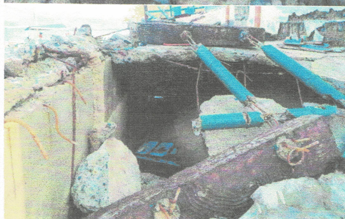
Photos of front hallway of Admin Building which was tear down by strong waves and the sand inside of it were washout
