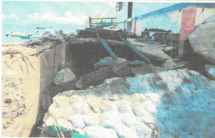
Photos of front hallway of Admin Building which was tear down by strong waves and the sand inside of it were washout
