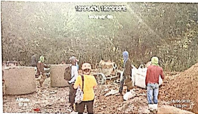
Workers within the quarry site observed making reinforced concrete pipe culverts (RCPC).
