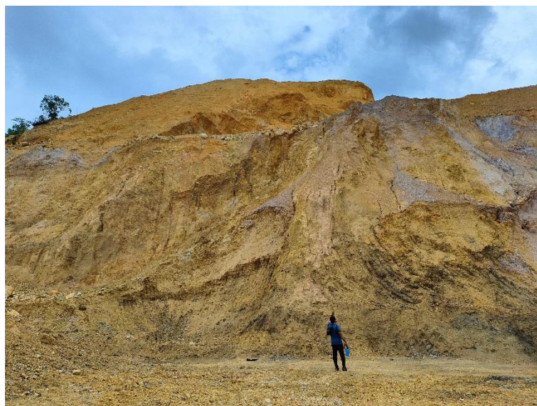
Photo 3. Majority of the slopes are comprised of thick, unconsolidated material.
