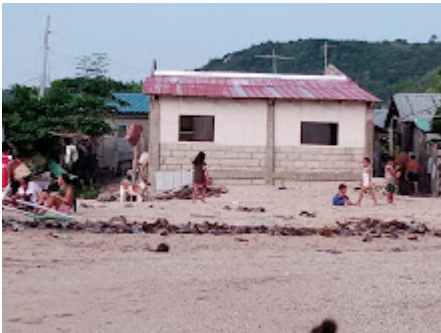
almost finish infrastructure in foreshore.jpg
