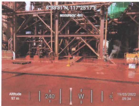
Bund walls surround the vessel containing chemical slurry.
