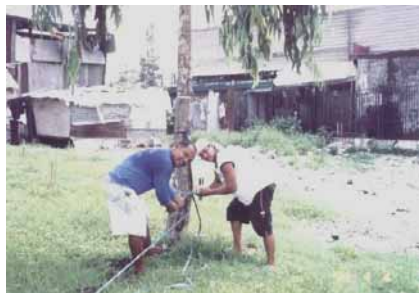
Fig. 6 Squatters living in the surrounding area were relocated and wastes were removed prior to the starting of the project.
