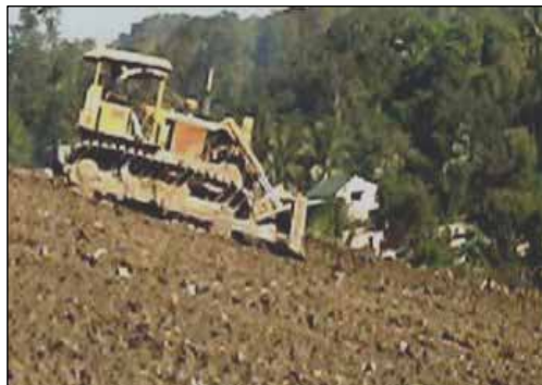
Fig. 21. At least 0.60 m of soil is being applied to the wastes at the end of each working day. The soil is then compacted to minimize the production of leachate, to control odor and to prevent the proliferation of flies, rats and other vermins.
