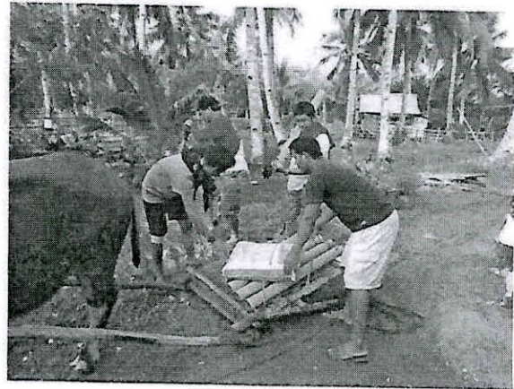
Hauling of Cemented PVC pipes, sand and cement for the footing using carabao in Brgy. Cheey, Busuanga.
