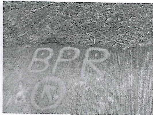
Spray paints was also use on paved roads to indicate the perimeter of BPR
