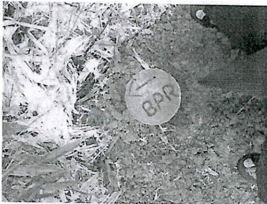
Directional arrow and BPR sign was engraved on top of the cemented PVC pipes
