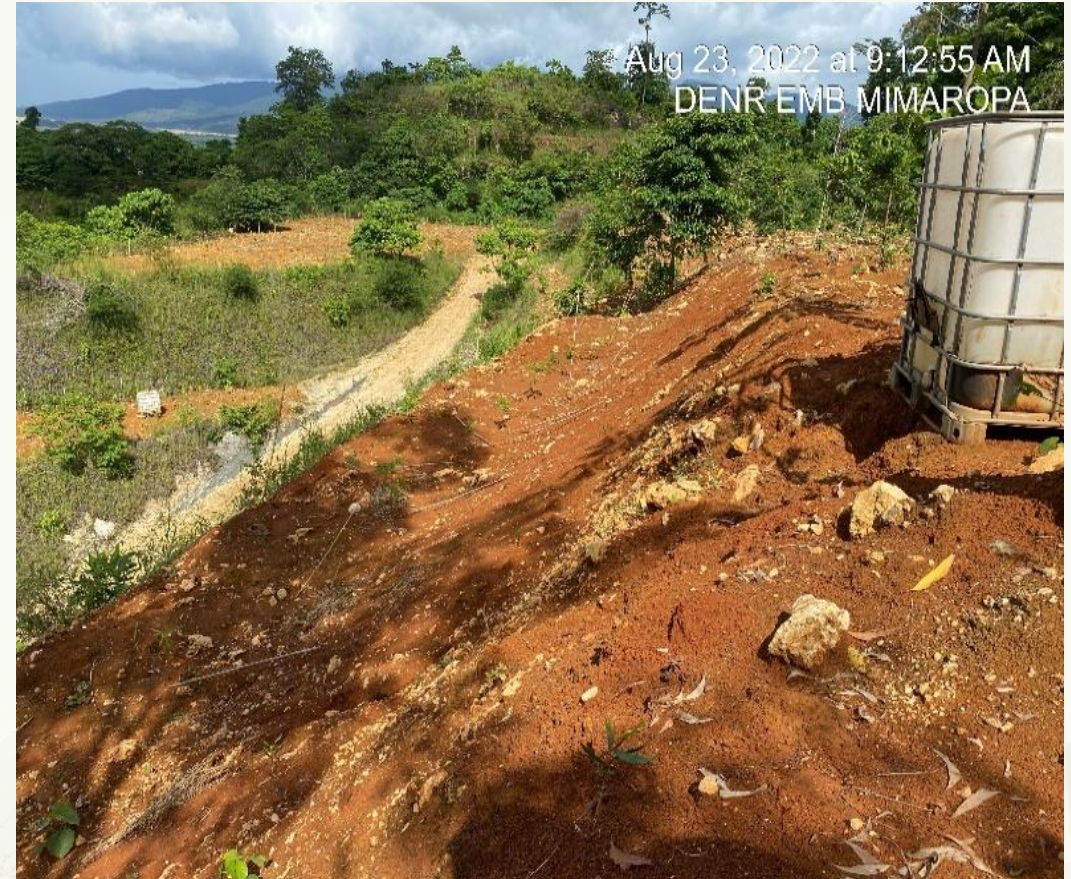
Bench recommended for revegetation to strengthen slope quality
