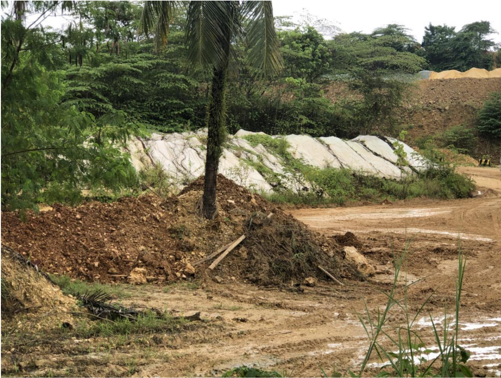
Photo showing a covered topsoil stockpile at the quarry area.
