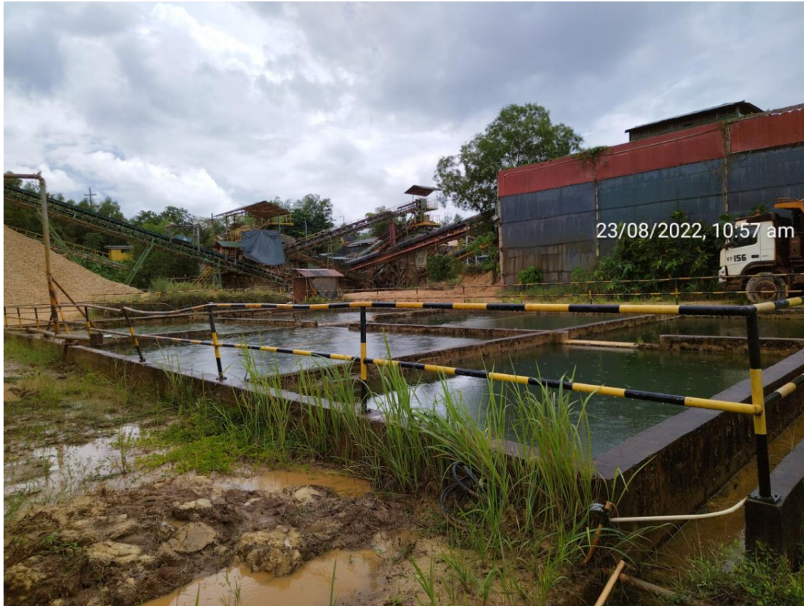
Photos of siltation pond at the crushing plant (left) and quarry area (right).
