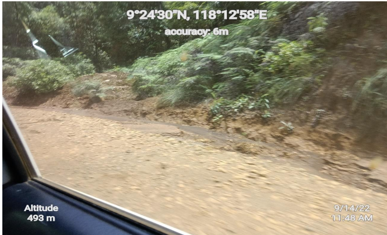
Photo 20. Observed accumulated silt at haul road drainage.
