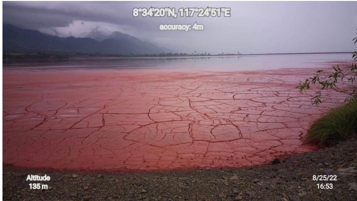
Photo 14 and 15. TSF 2 inspection. The tailings deposits is at 79.3 masl at the time of inspection.
