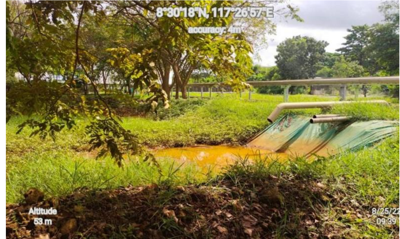
Photo 11 and 12. MMT Members inspects the Earth pond silt collector which drains the silt from the main silt collector. No signage provided.
