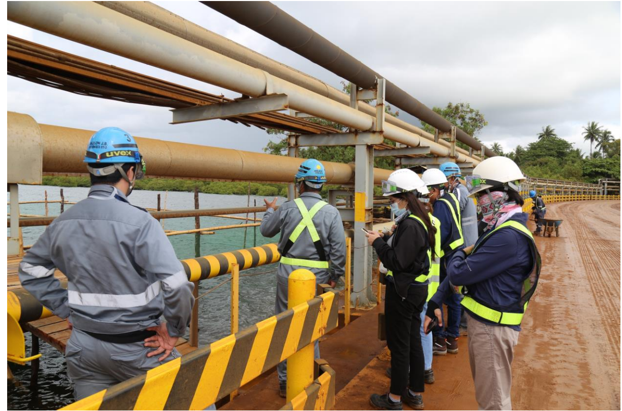
Photo 10. Pipes (upper 2) discharges treated wastewater from the plant and replenishes caustic soda, sulfuric acid and methanol used in the HPAL process.
