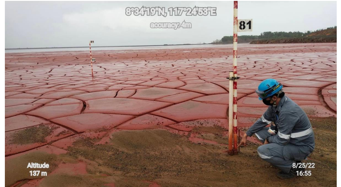
Photo 14 and 15. TSF 2 inspection. The tailings deposits is at 79.3 masl at the time of inspection.
