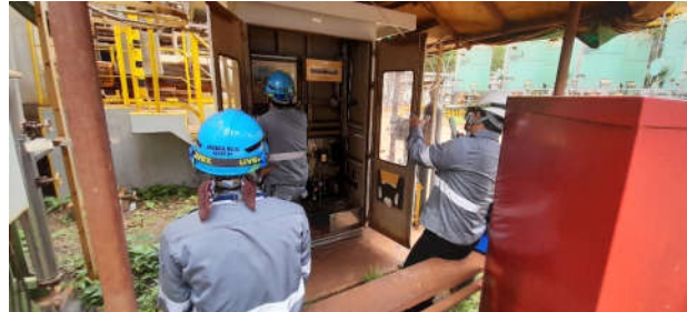
September 14, 2022 Cylinder Gas Audit was conducted. Witnessed by Engr. Mark Angelo Rogel of EMB MIMAROPA. All CEMS reading are accurate base on the CGA result.
