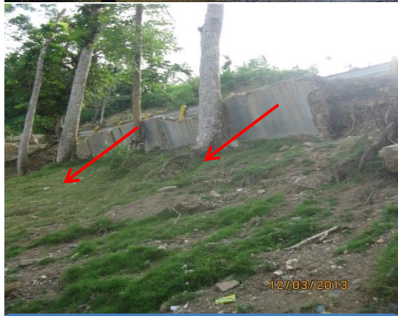
Tilting of fence/walls
