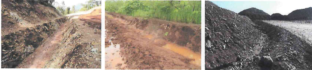
Figure 8. The constructed canal for run-off diversion
