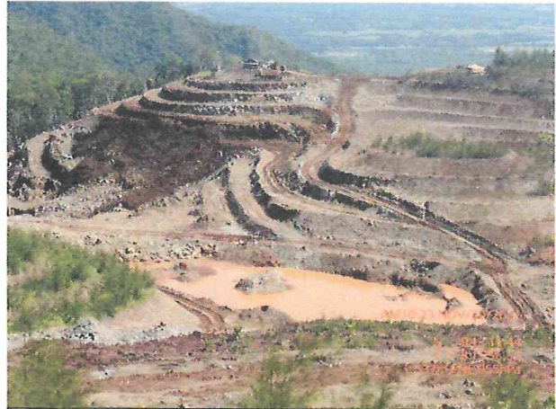
Figure 3. Block A Rehab 7 benching
