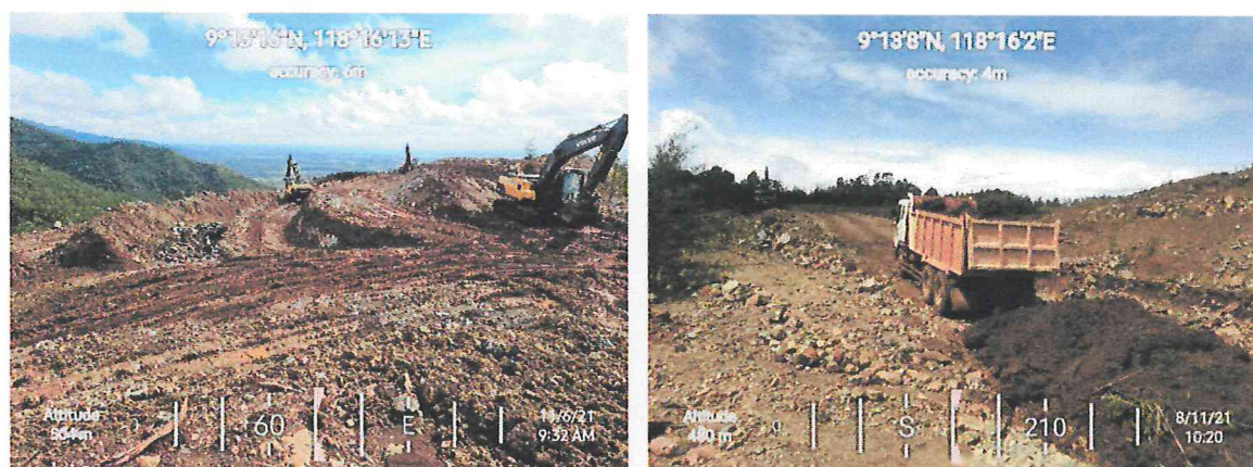
Figure 5. Contouring and Topsoil Matting in Block A Rehabilitation areas
