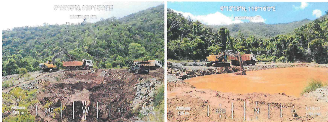
Figure 12. Desilting of Silt Control Structures
