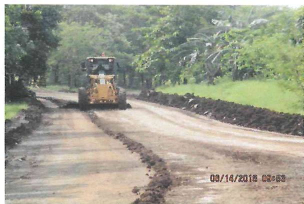
Figure 13. Scraping of Hauling Road
