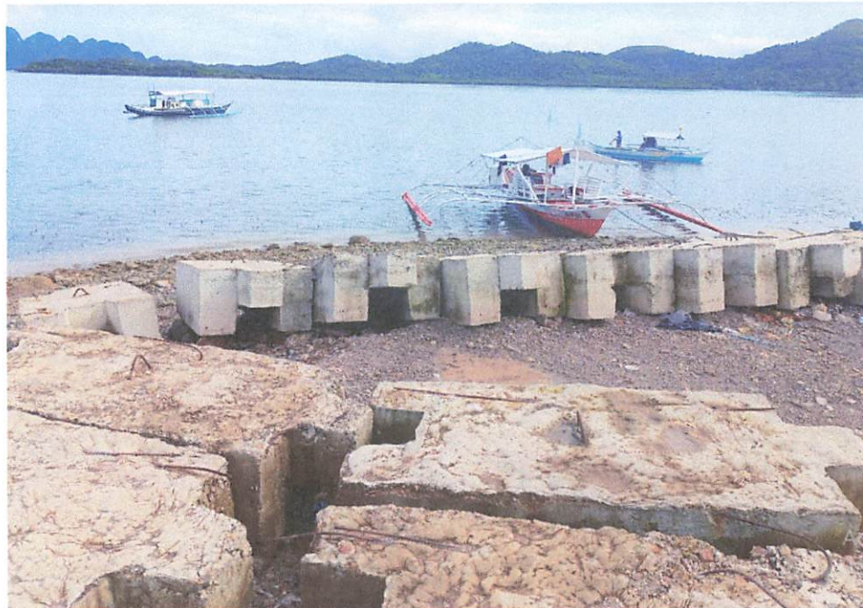
Figure 11. Cement post left unused for the construction of the seawall
