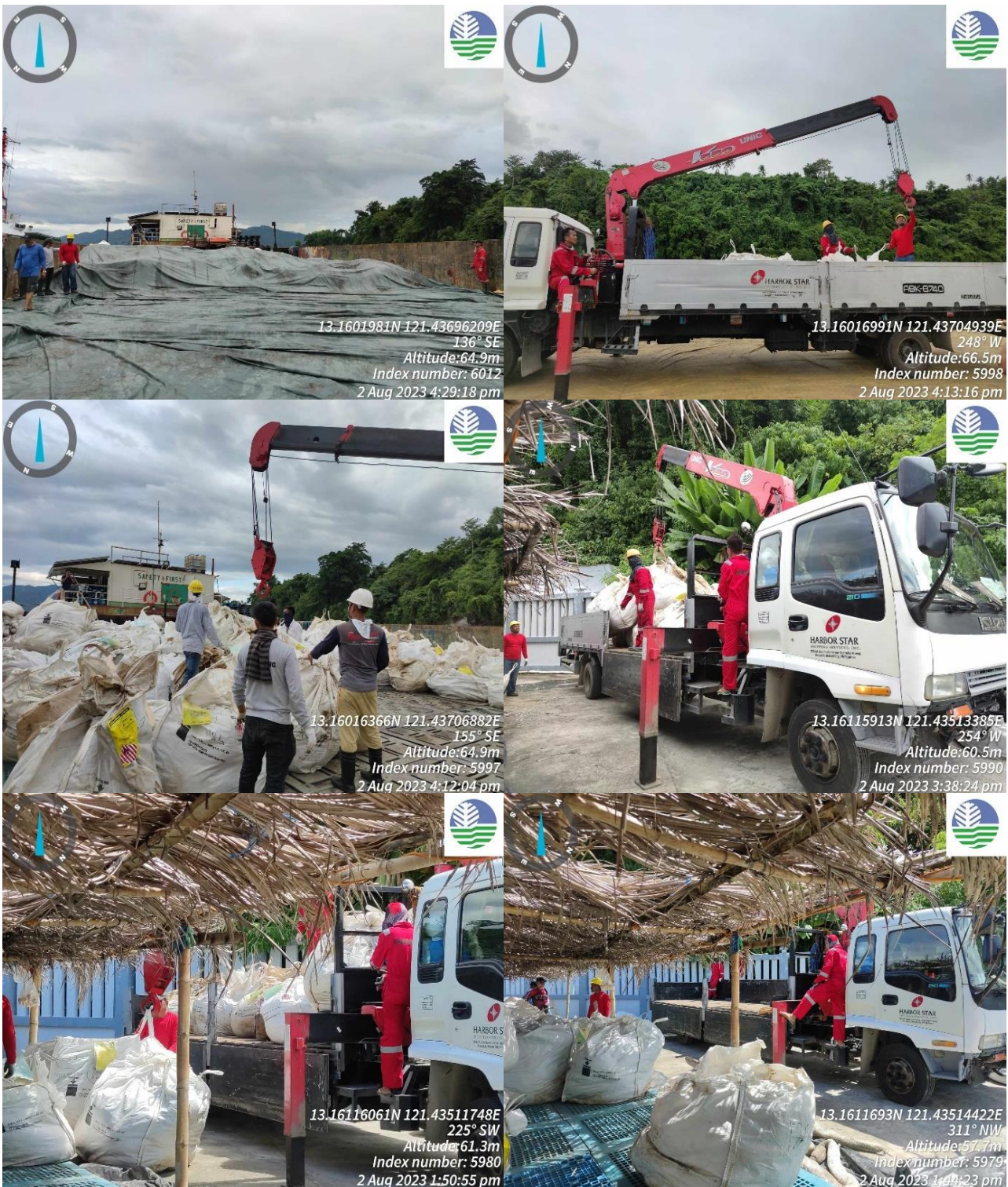
August 2, 2023 - Tonner bags were placed atop rows of palette with another layer of tarpaulin and sorbent pads below to prevent leakage. Sorbent booms were also placed around the rows of palette for added protection.
