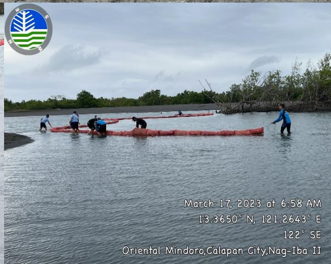
March 17, 2023 - Installation of improvised spill booms at Sitio Duluhan, Brgy. Melgar B, Naujan
