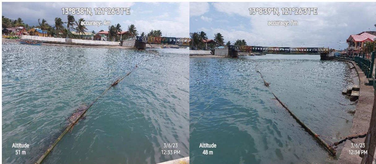
March 6, 2023 - Installation of improvised absorbent boom in Casiligan River, Pola Oriental
