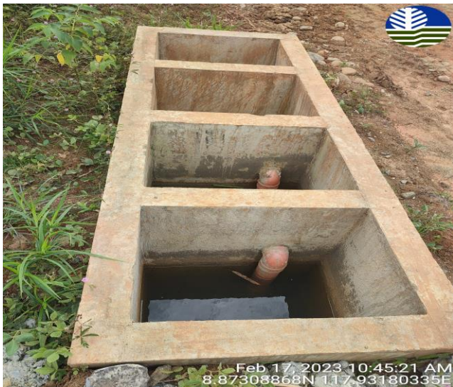
5 units of Oil and Water Separator.
