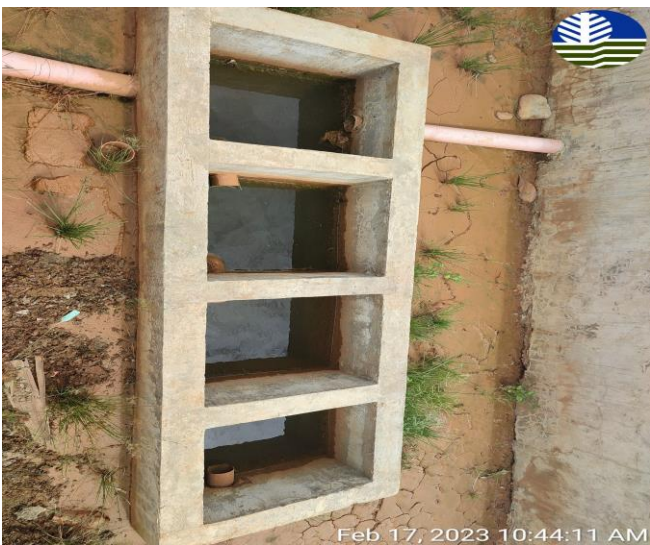
5 units of Oil and Water Separator.
