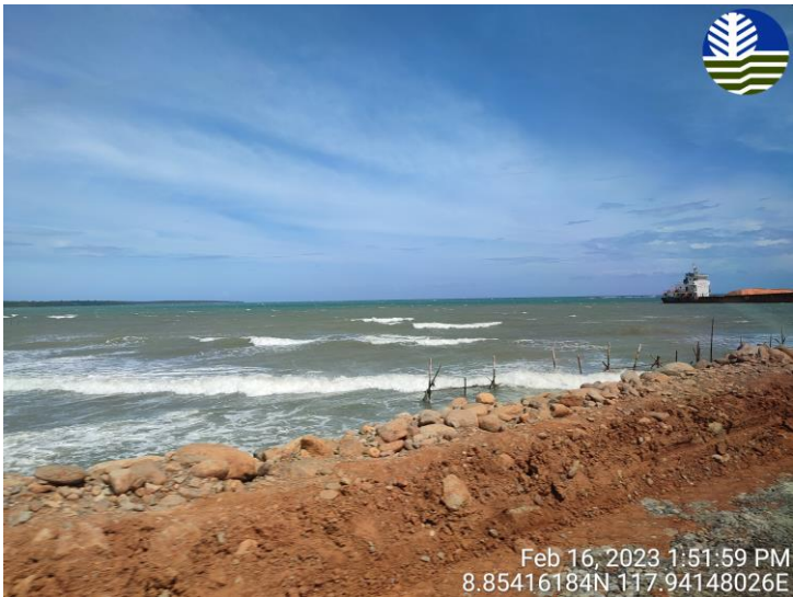
Installed Silt fence that needs maintenance and repair.
