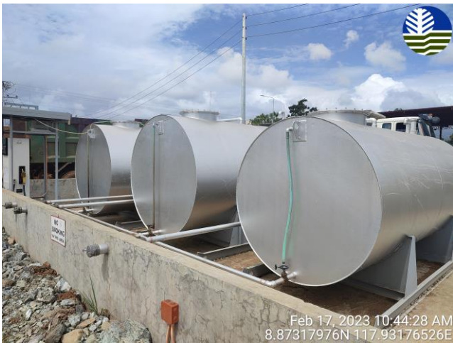
Fuel tanks with a total of 94 KL located at mine camp.
