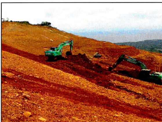
Bench/slope correction and re-soiling works
