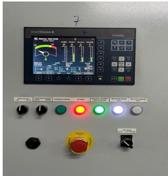
Figure 11. GENERATOR SET ONTROL PANEL
