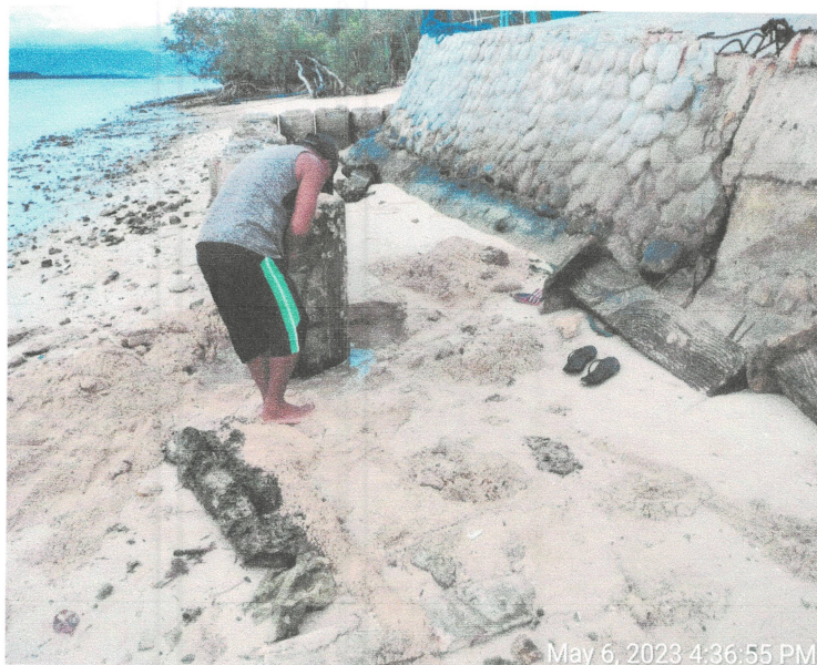
Photos during the placement of culvert in front of Snake Island Administrative Building
