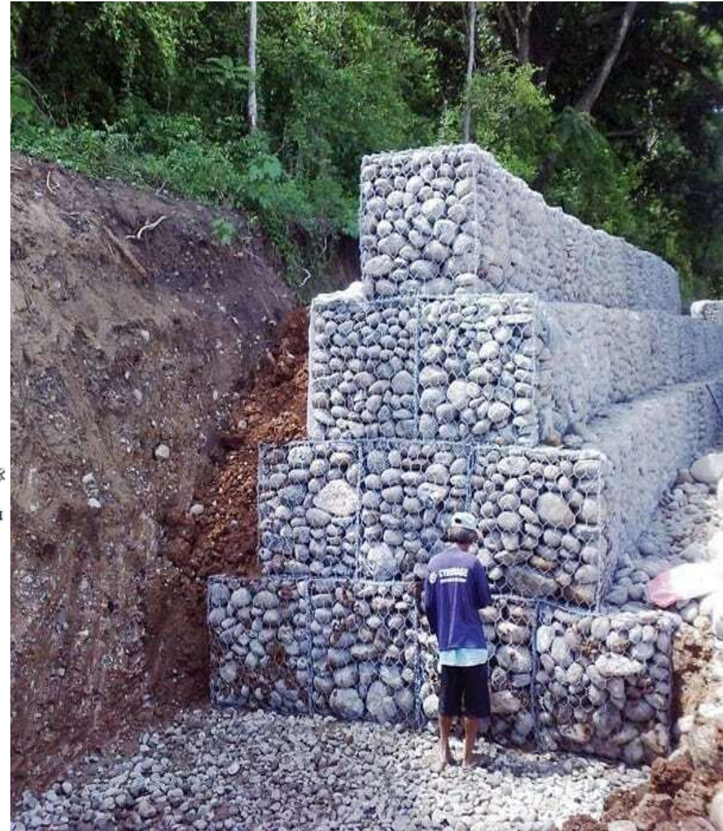
Figure 5_Gabion Wall to protect river banks from erosion and flooding hazard to the community and their crops.
