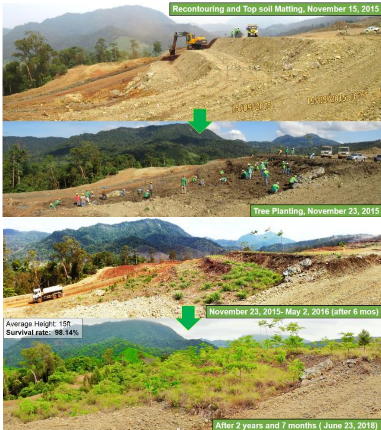
The sequence of Mined-out Rehabilitation Illustration
