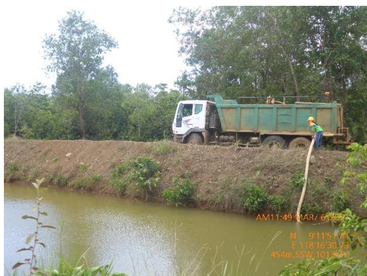
Figure 8. Siphoning of Water for Road Sprinkling
