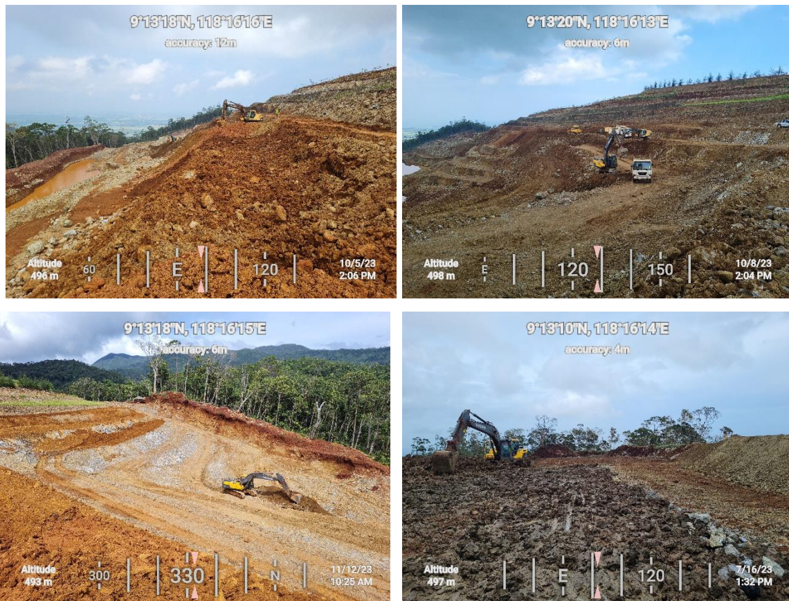
Figure 12. Backfilling, Recontouring and Topsoil Matting in Block A
