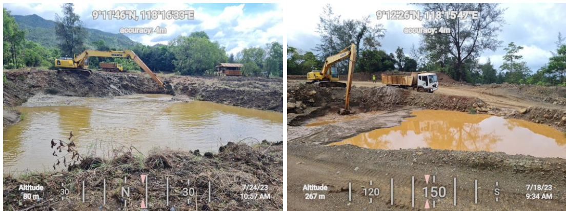
Figure 26. Desilting of Silt Control Structures
