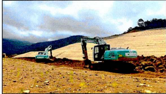
Bench/slope correction and re-soiling works
