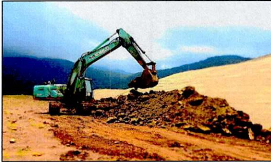
Bench/slope correction and re-soiling works
