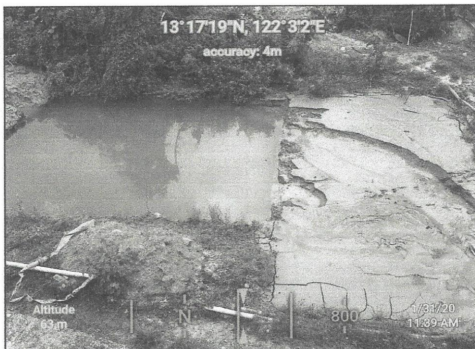
Figure 7. The tailings pond of Palatino Trading overflowing with sludge materials
