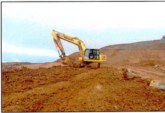
Land preparation (Slope Stabilization–bench correction works)
