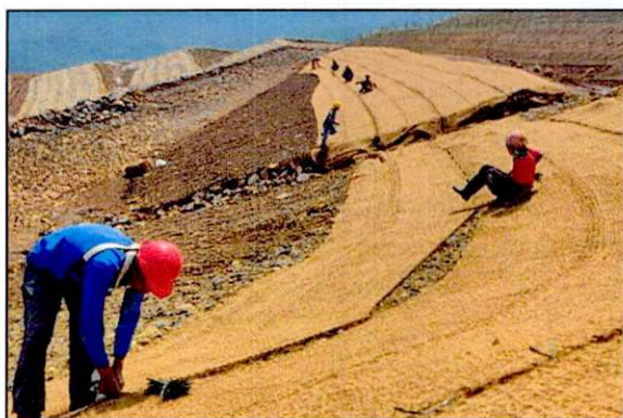
Installation of Coco-coir net in Mine Rehabilitation areas
