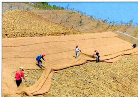
Installation of Coco-coir net in Mine Rehabilitation areas
