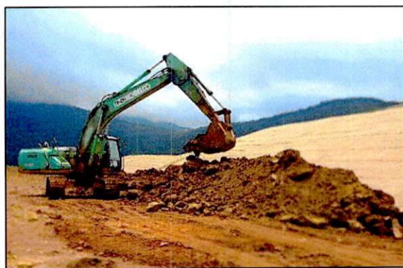
Land preparation (Slope Stabilization–bench correction works)
