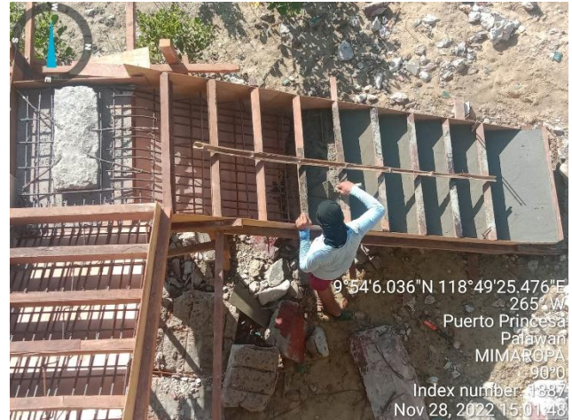
Photos during the helipad's staircase construction
