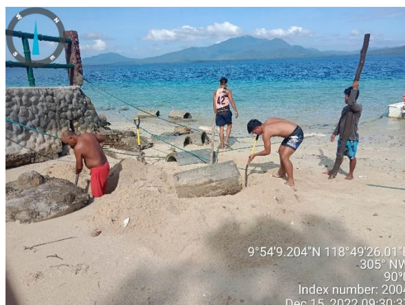
Photos during the installation of the culverts in their original location in front of the administrative building as a breakwater
