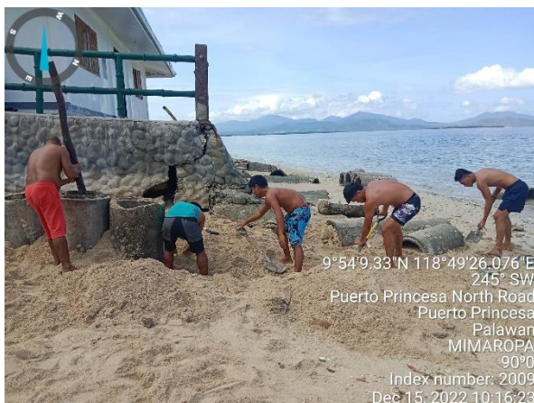
Photos during the installation of the culverts in their original location in front of the administrative building as a breakwater
