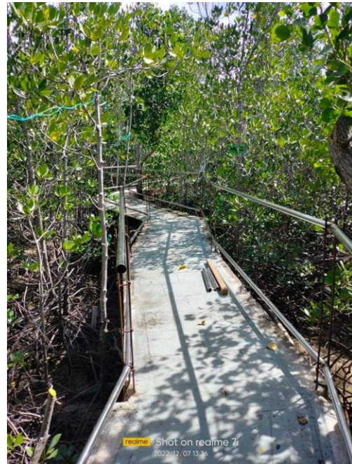
Photos during the new stainless steel railings being installed and the boardwalk being repaired
