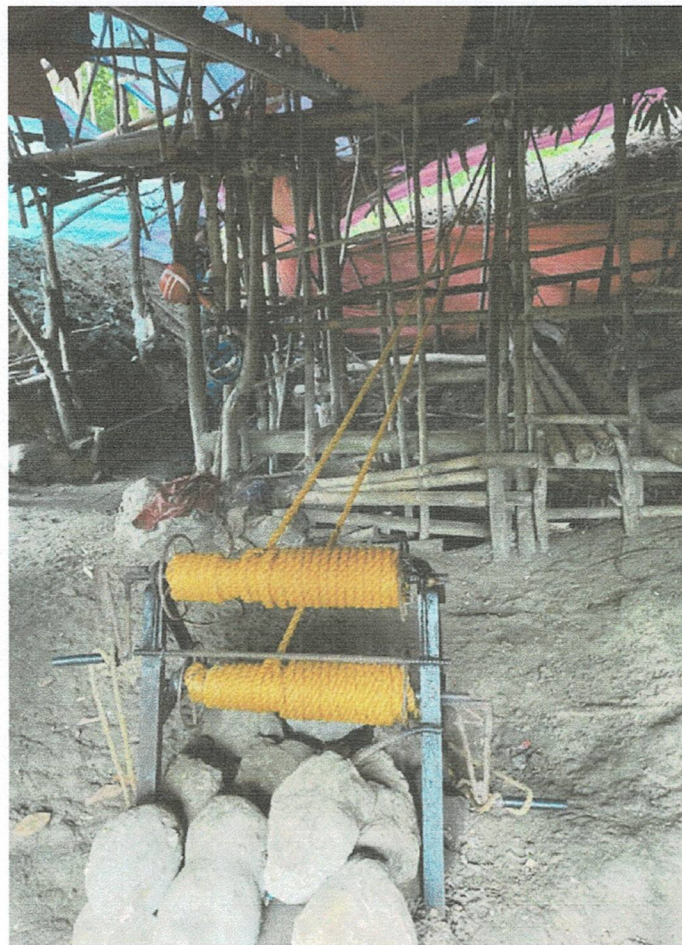
Entrance of the pit. Timber framework noted on site providing stability to the pit walls.
