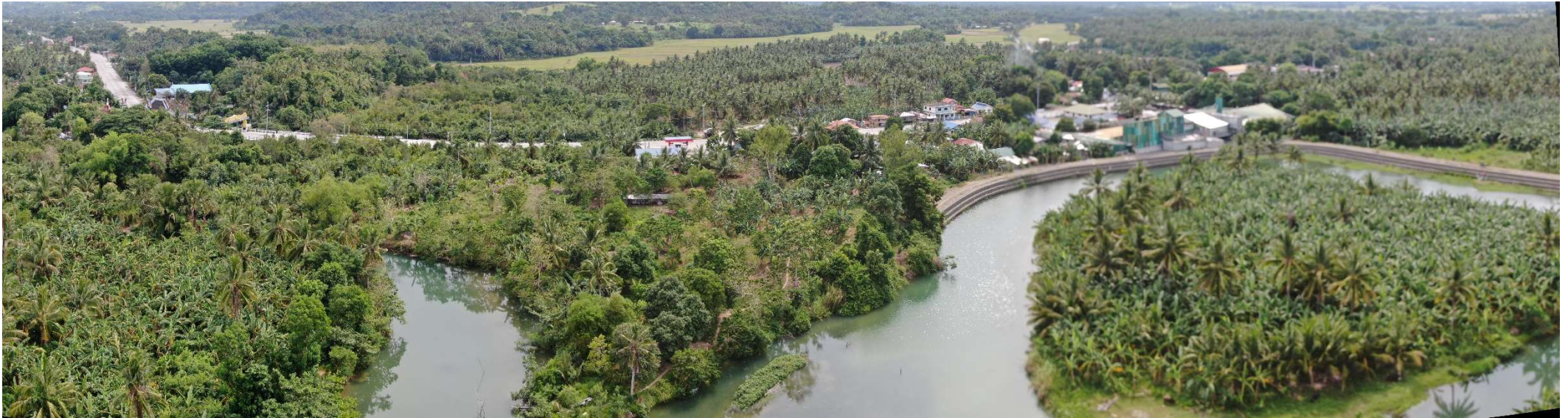
Photo No. 3_Panoramic view of the SUMAGUI RIVER using DJI Mavic 2 Zoom Drone showing the contoured stream where some portions of its bank are protected with gabion walls to prevent overflow or flooding.
