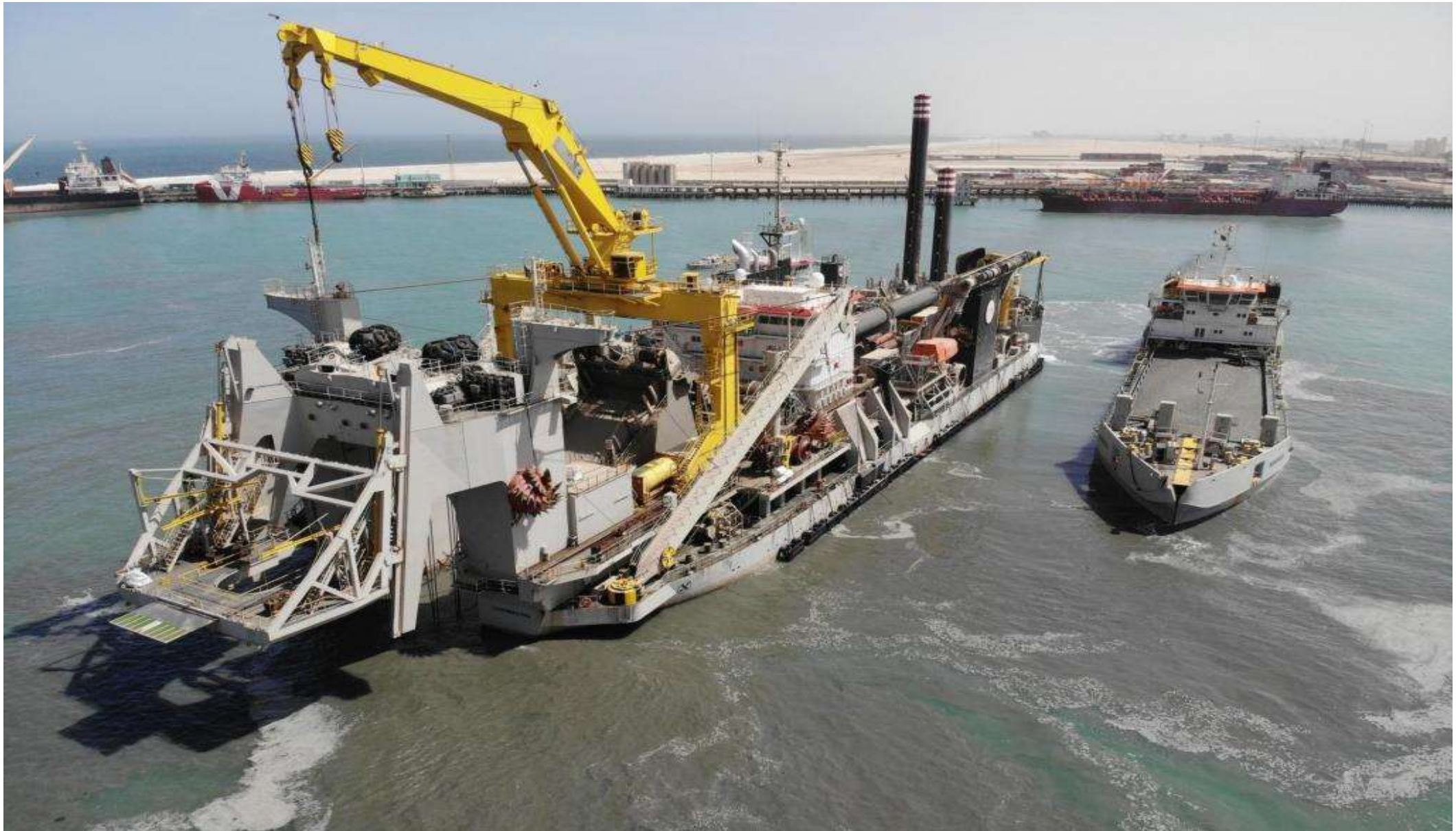
Figure 3_Cutter Suction Dredger and barge.
