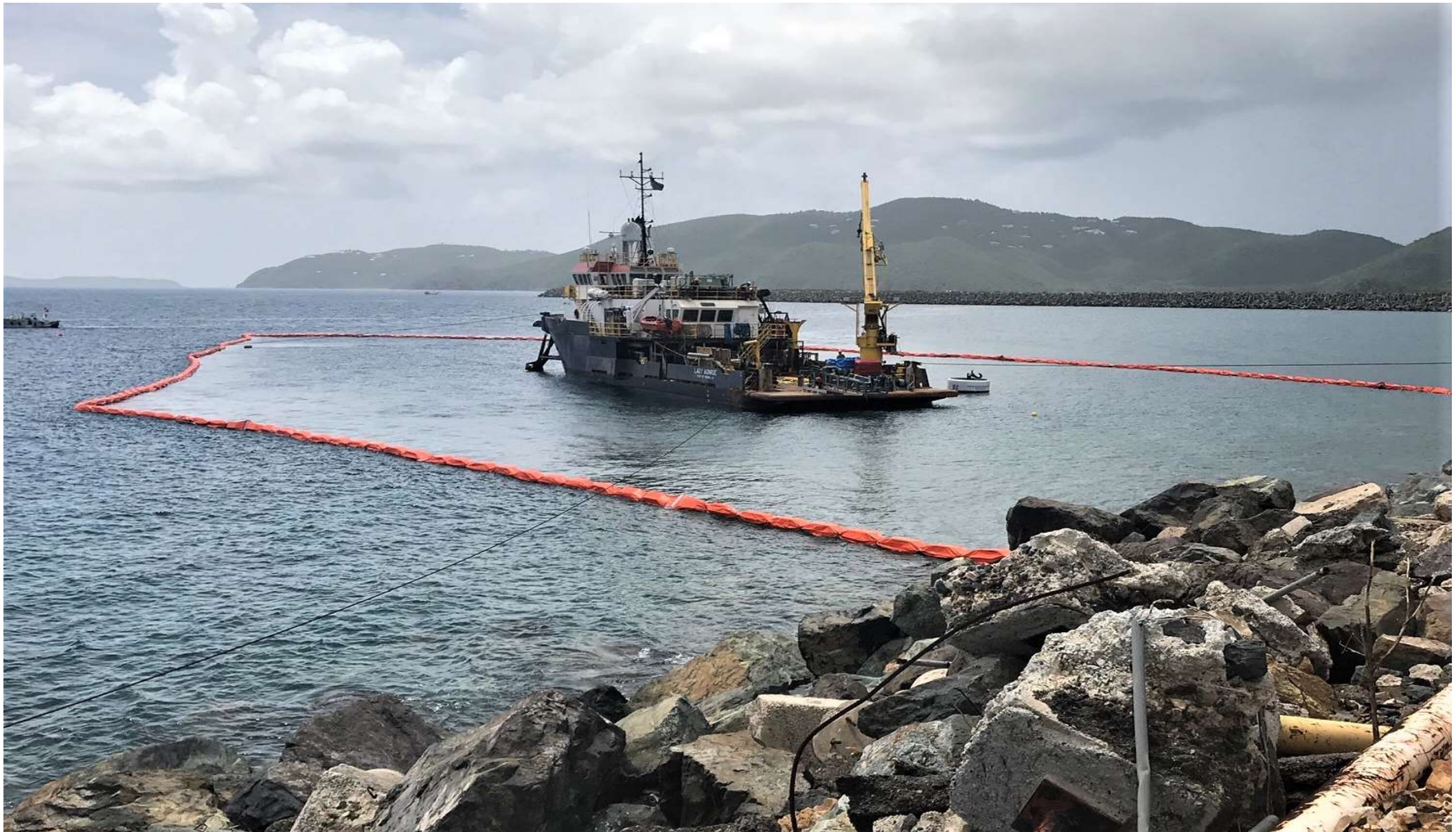
Figure 4_Sample of Silt Curtain installation to contain disturbed water from polluting other parts of Tablas Strait that can damage or destroy marine habitat.
