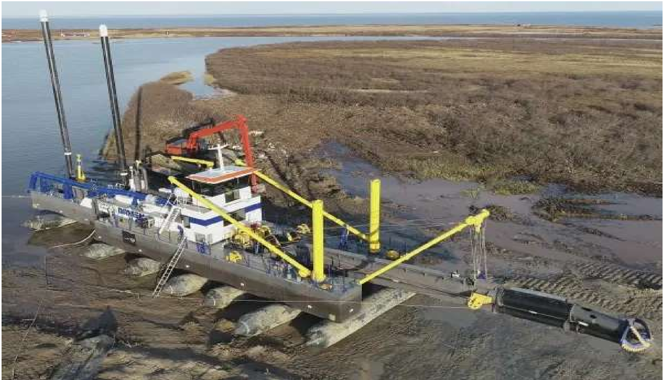
Figure 2_Cutter Suction Dredger – Damen CSD 250, showing 2 spuds to position the dredger steadily.
