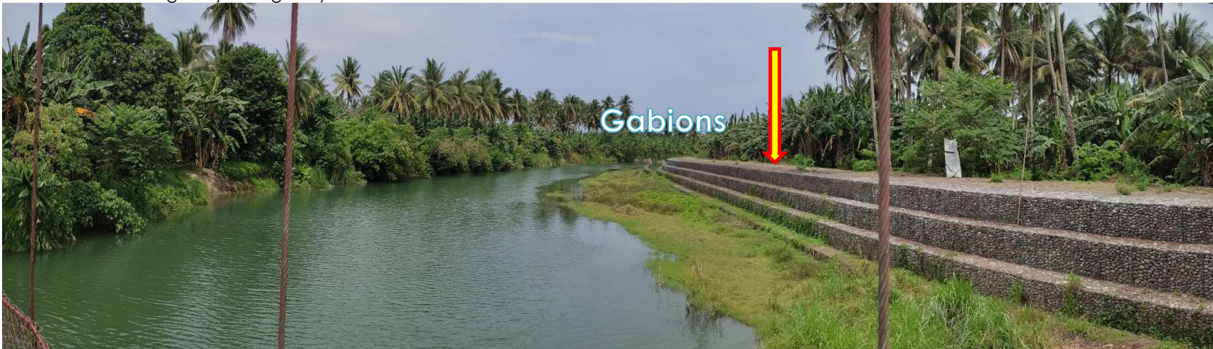
Photo No. 5_Panoramic view showing western section of SUMAGUI RIVER equipped with gabions for protection from flooding hazard and erosion.
