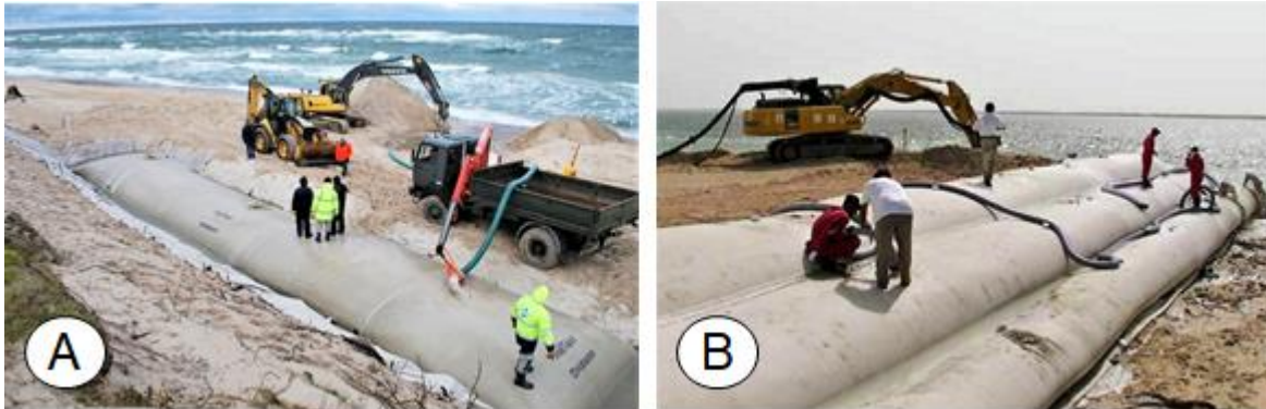
Plate 2.1.3: Placement of Sand Bags and Geo-Tubes
