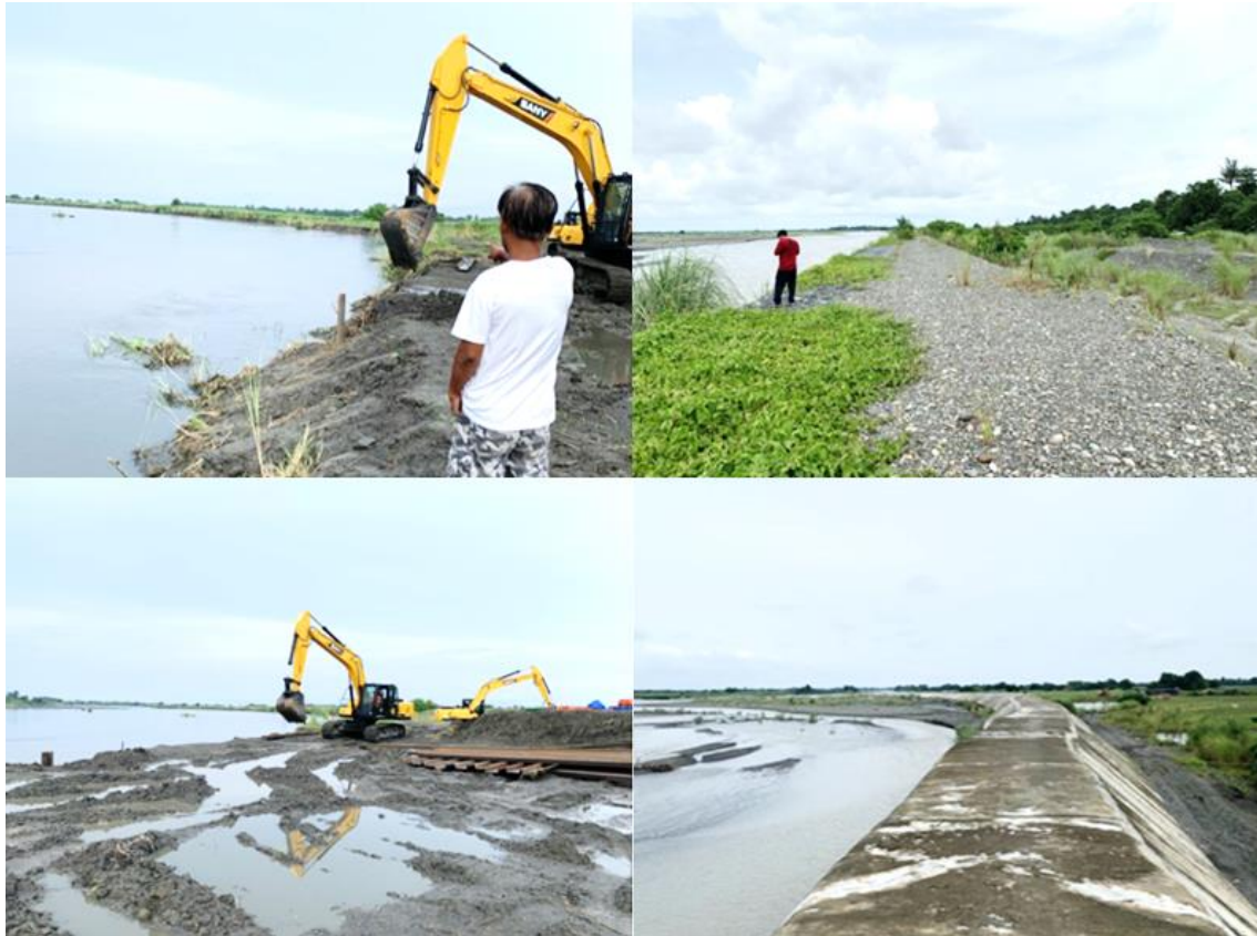
Plate 2.2.7: Existing Bank Protections and those Under Construction for Amnay and Patrick Rivers Consisting of Sheet Piles, Embankment and Gabion Walls
