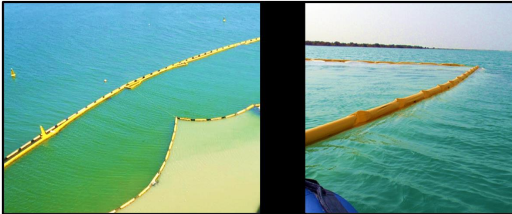
Plate 1.4.1: Silt Curtain (Barricade) to Separate Sludge from Adjacent Water Bodies Surrounding the Offshore Dredging Area
