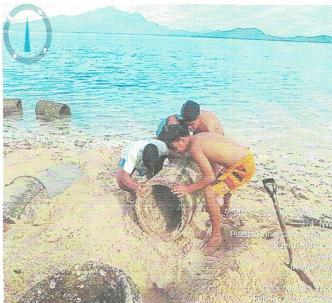
Photos during the placing of culvert in front of Snake Island admin building
