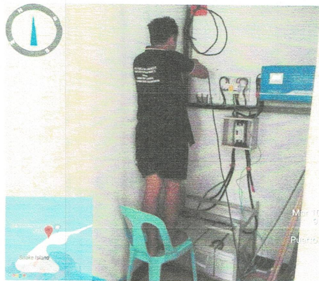
Photos during the installation of solar charger controller and re-wiring of electrical system
