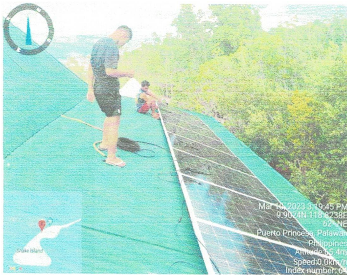
Photos during the installation of solar charger controller and re-wiring of electrical system
