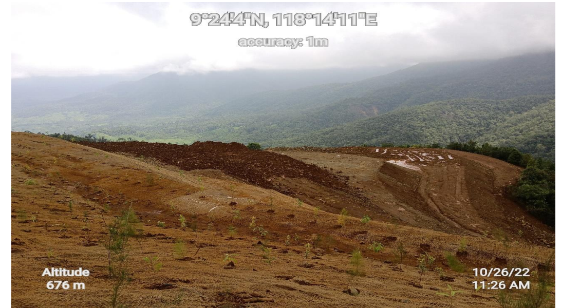
Photos 4 & 5. On-going land preparation (topsoil matting & slope benching) observe at Area 12.
