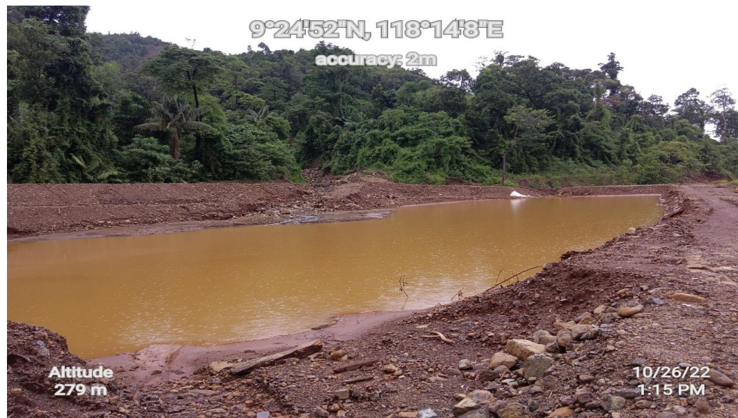
Photos 15 & 16. First compartment of the series of siltation ponds at kilometer-7 (left) which ultimately drains to BSW-1 (right), the discharge point of BNC.
