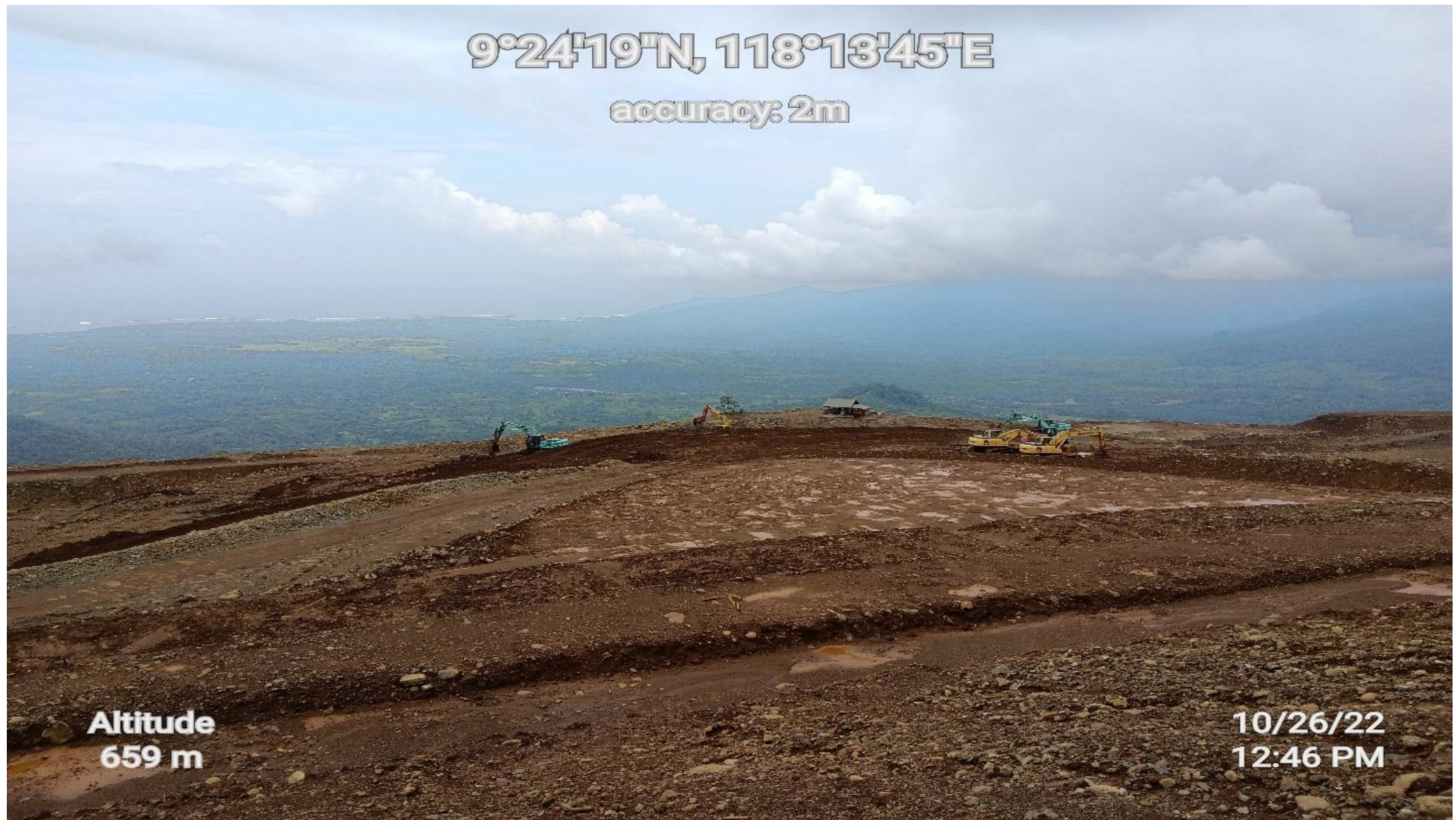
Photo 4. On-going land preparation (top soil matting & slope benching) observed at Area 16.
