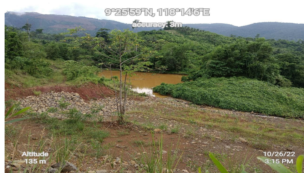
Photos 15 & 16. First compartment of the series of siltation ponds at kilometer-7 (left) which ultimately drains to BSW-1 (right), the discharge point of BNC.
