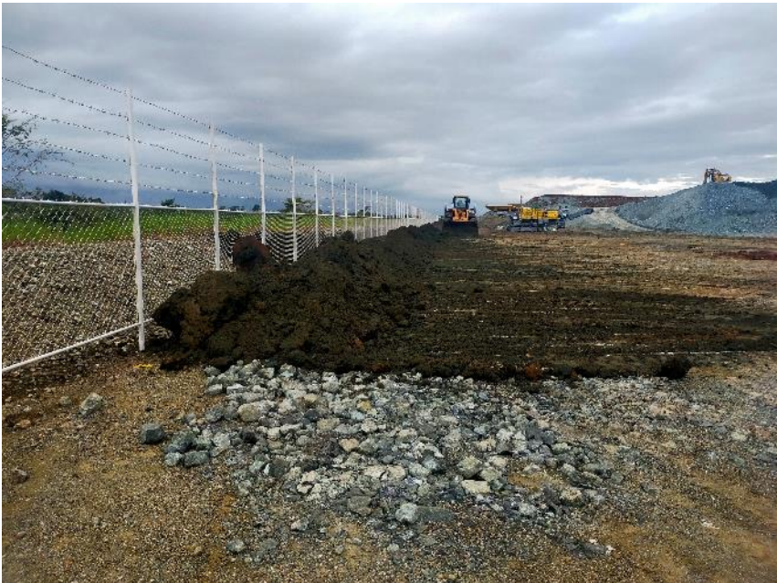
Top Soil Overlay. Around 0.5 meter thickness
