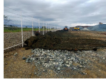
Top Soil Overlay. Around 0.5 meter thickness
