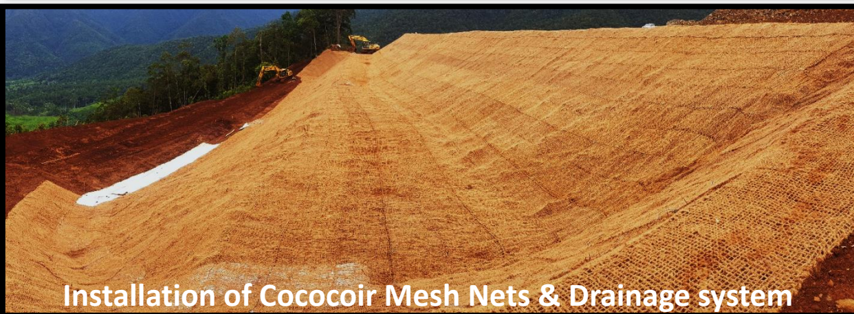
Slope Stabilization, Bench Correction, Re-soiling
